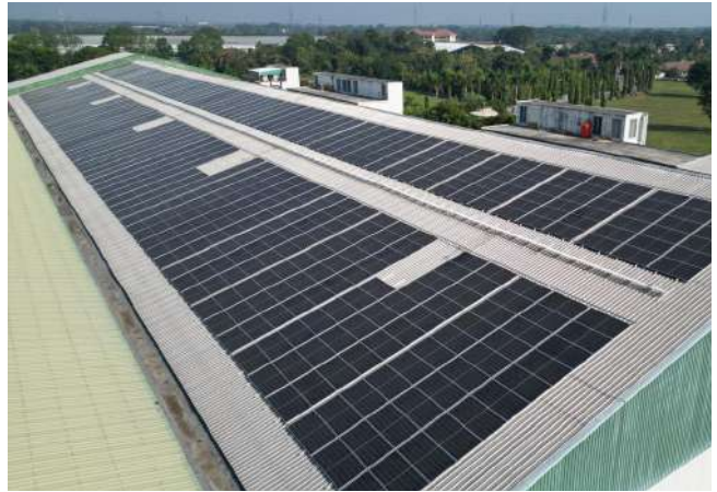
Installation of solar panels at the roof top of spun yarns factory Pemasangan panel surya di bagian atas atap pabrik pemintalan benang
